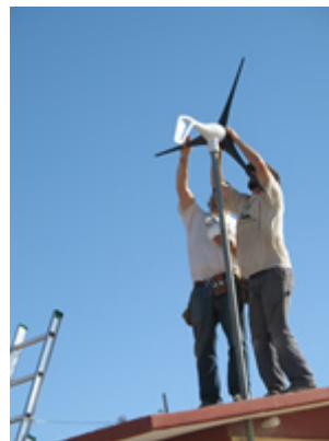
Wind mill Installation in Laguna San Ignacio
