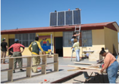
Solar panel installation in Laguna San Ignacio
